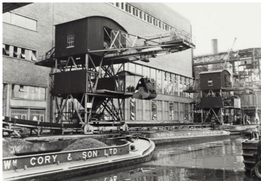
Figure 1: Hackney Power Station, Millfields 1950-69
