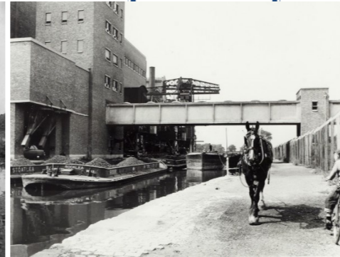
Figure 4: Hackney Power Station, Millfields 1950-69
